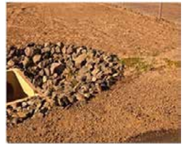
Environmental silt fencing and rock check dams
