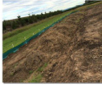
Environmental silt fencing and rock check dams
