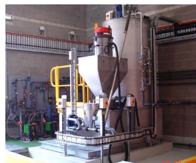
(L) HYDRATED LIME SLURRY PUMPING SYSTEM AND (R) POLYMER BATCHING AND DOSING SYSTEM
