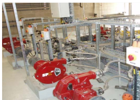
(L) HYDRATED LIME SLURRY PUMPING SYSTEM AND (R) POLYMER BATCHING AND DOSING SYSTEM
