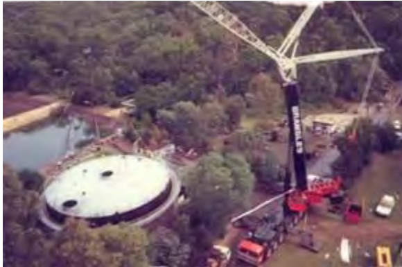
Digester gasholder installation
