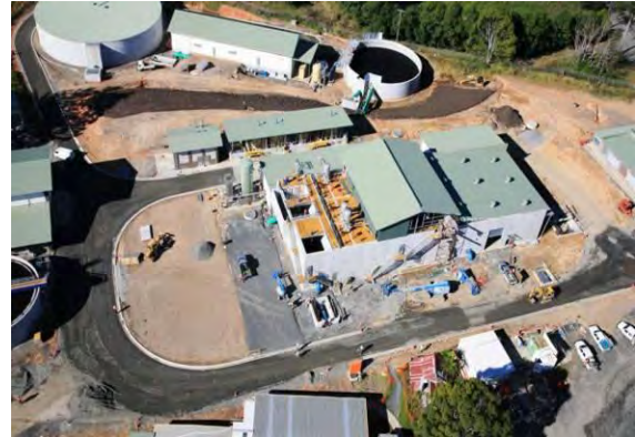
Karangi Dam WTP
